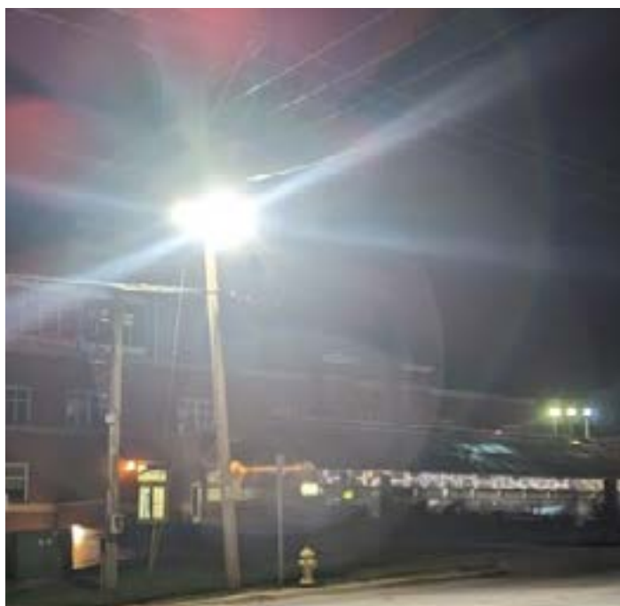
Figure 3: Badly designed light fixtures are responsible for causing glare. Glare impairs vision and can reduce both pedestrian and driver safety. Note the contrast between the brightly lit area right under the light, and the sudden transition to relative darkness toward the bottom right. A pedestrian attempting to cross the street from the far sidewalk, which is shrouded in darkness, is at risk of being invisible or only partly visible to drivers.
